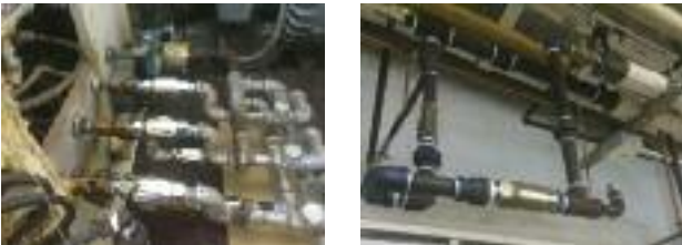
Apollo Trap Installation
